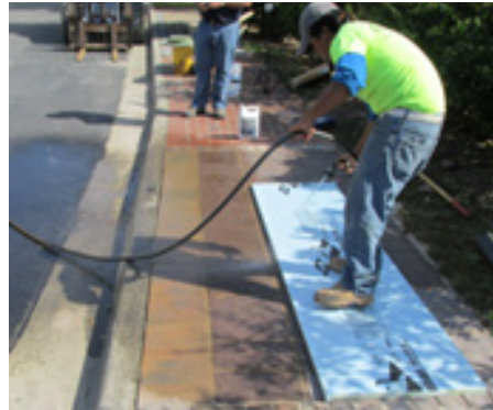
Wet down per commercial paver cleaner instructions
