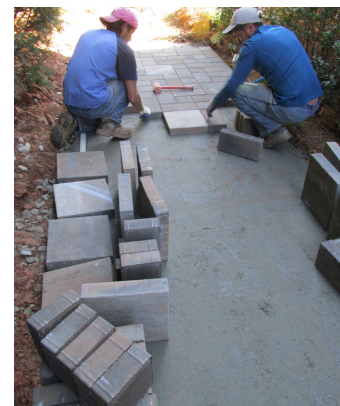
Notice how pavers are stacked on their sides or single stacked
