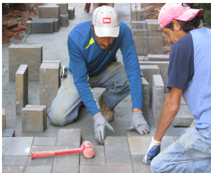
Use a rubber mallet for paver installation.
