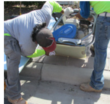
A clean neoprene pad protects textured and dark color pavers from surface scuffs
