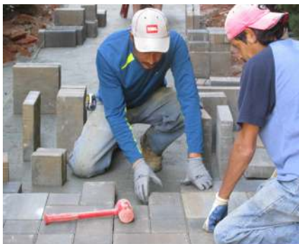
Use a rubber mallet for paver installation.
