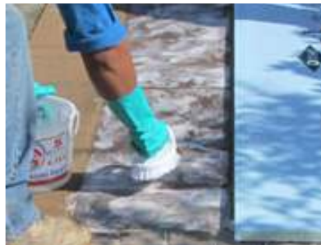
Scrub with commercial paver cleaner and soft brush
