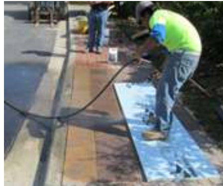
Wet down per commercial paver cleaner instructions
